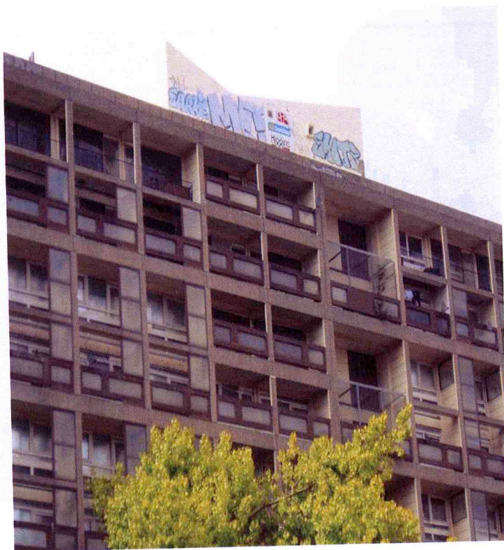
High rise tower block – Lambourne House
